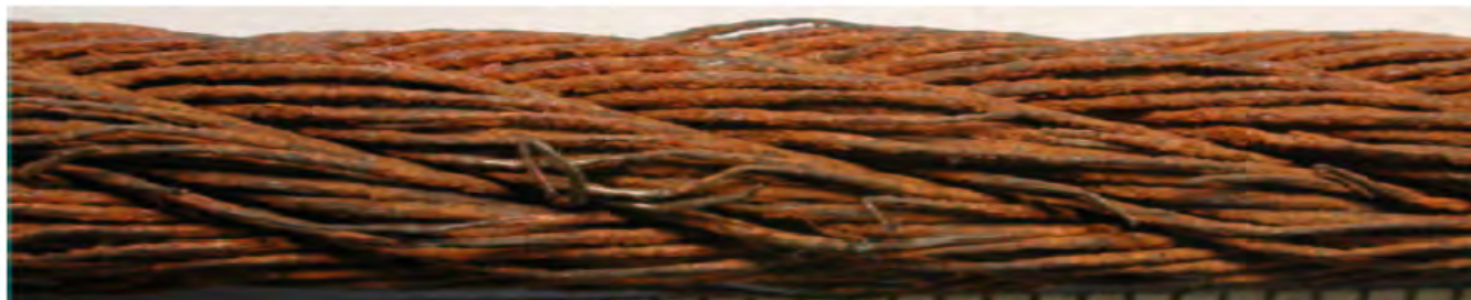
Figure I.3 — Surface heavily pitted and slack wires Discard immediately, i.e. 100%
