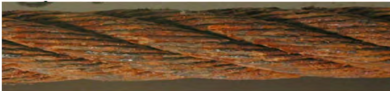
Figure I.2 — Wires rough to touch - general surface oxidation of the wires Rating: 60% towards discard
